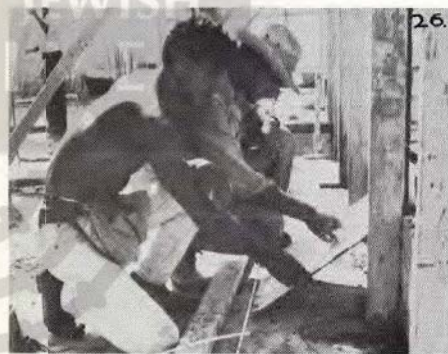
Last year, these home builders were in the crew of an Israeli tank speeding through Sinai. Today, they begin to erect the walls of a clinic in one of the country's 21 new development towns. Skills like these are learned at ORT schools supported by contributions to the 1969 United Jewish Appeal Emergency Fund.
