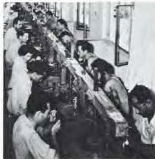
Skilled workers cutting and polishing industrial diamonds, which are now Israel's largest export.
