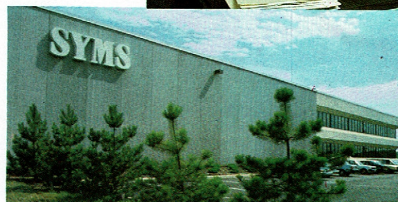
Distribution Center and Executive Offices in Lyndhurst, New Jersey. 100,000 square feet. Open August, 1981.
