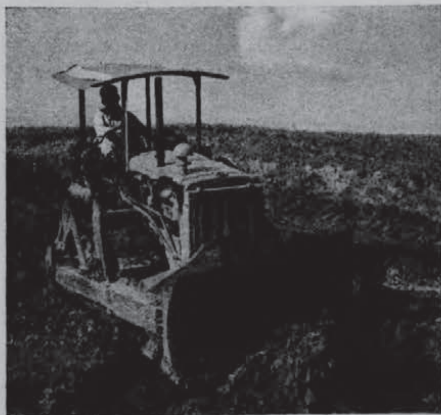
Patching up Eroded Soil. Tractor with angledozzer filling in crevices
