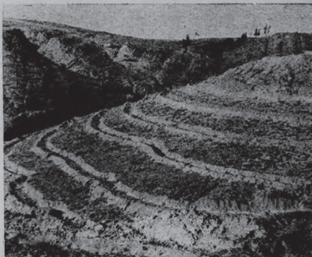
Erosion Control at Ruhama : Terraces and Flat Ditches along contour lines.
