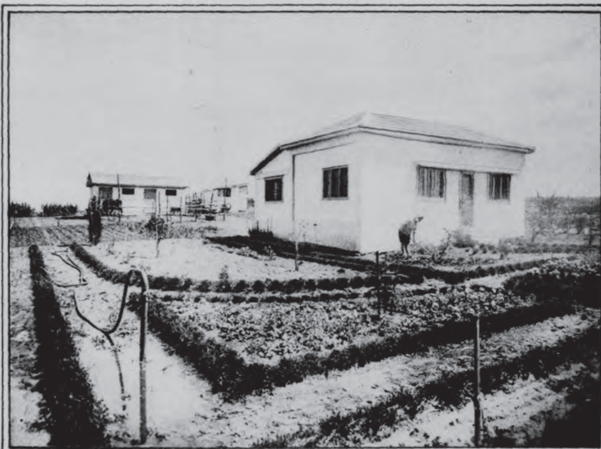
A TYPICAL JEWISH FARMSTEAD IN BENJAMINA: HOME OF A NEW IMMIGRANT. Who With Funds Supplied by a Mortgage Bank Has Built a House and Is Engaging in Truck Gardening and Poultry Raising.
