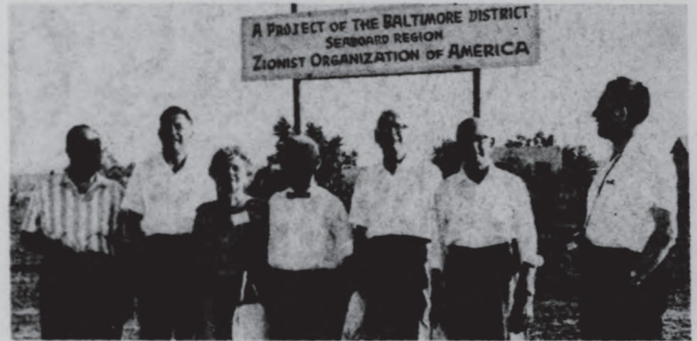
GROUND-BREAKING for school building project of the Seaboard Region.
