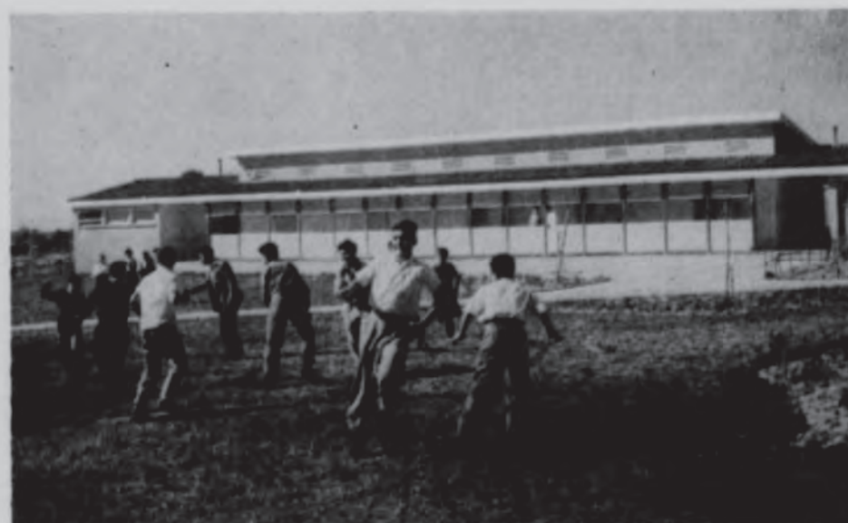
FOSTER DORMITORY consists of two similar wings (of which one is seen here) connected by an open-air patio. The dormitory is a gift of Mr. and Mrs. Joseph Foster of Leominster, Mass. It has nine rooms for students, a spacious club room and a small apartment for the supervising instructor. The landscaping has just started.
