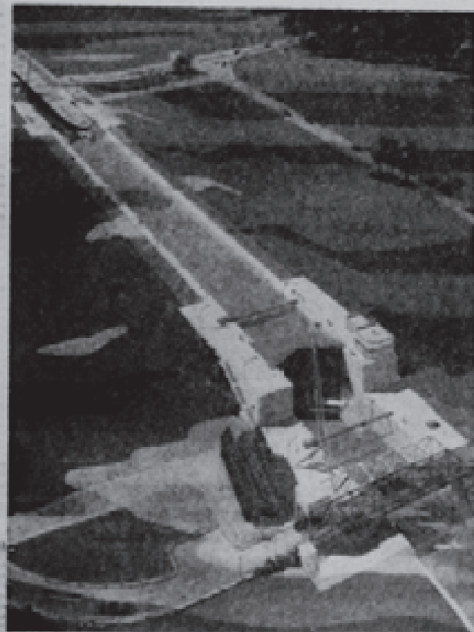
SKETCH shows how traffic over Grasse River Lock will be uninterrupted while vessels pass through. Traffic is routed to bridge at bottom while bridge at top is blocked.
