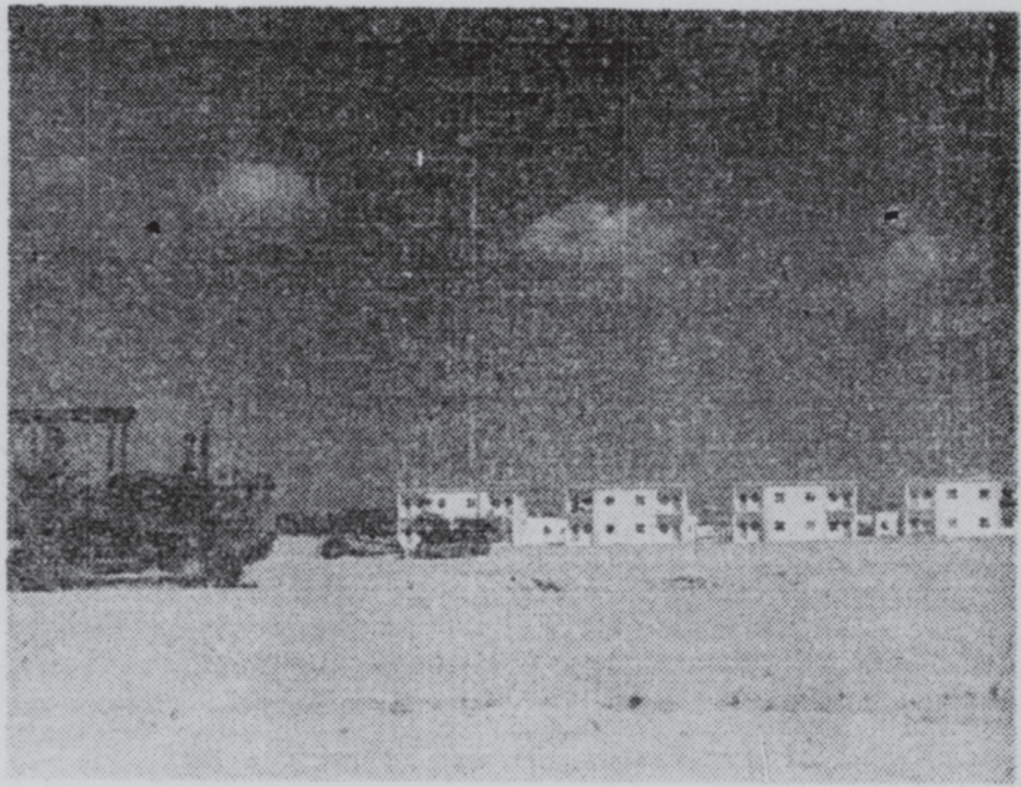
At Kiryat Haim near Haifa. Tractors levelling the sand-dunes for the construction of new houses.
