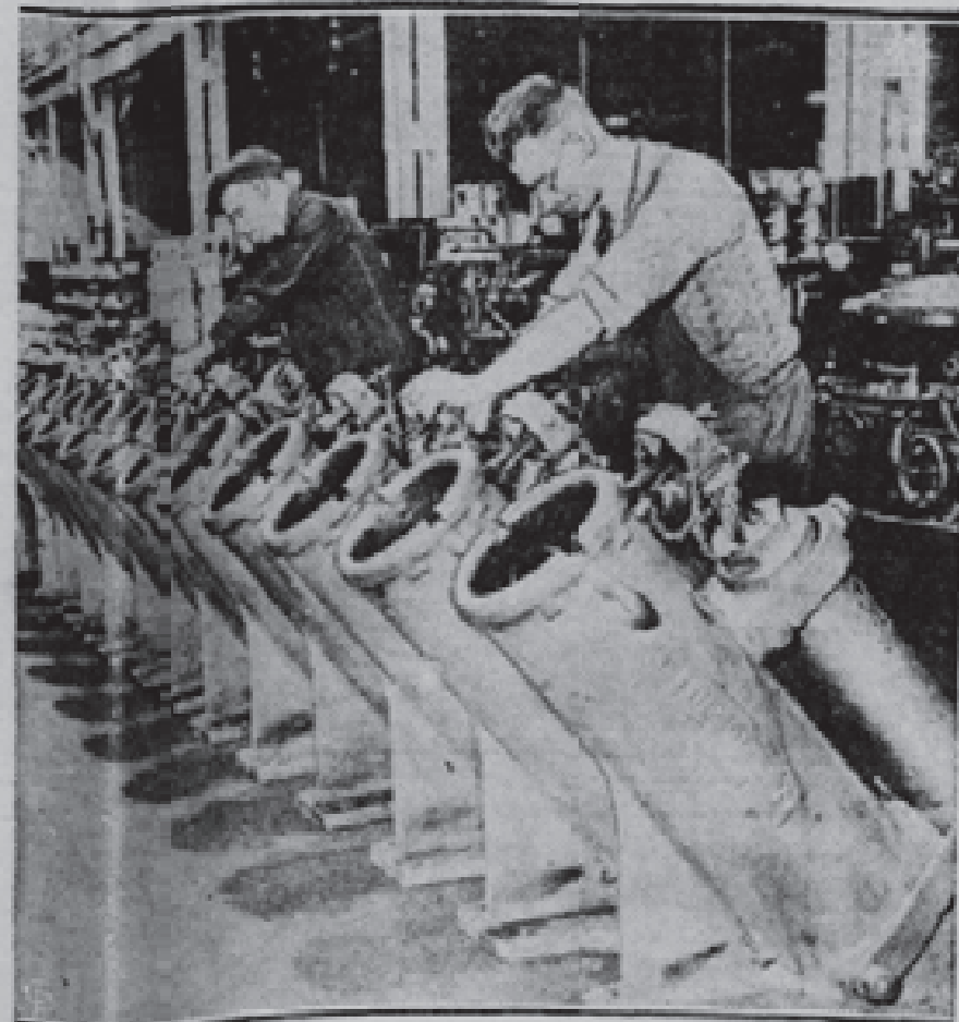
Above is pictured a battery of depth-charge throwers awaiting inspection in a British naval plant. Officers and crew of a raiding submarine have learned to fear this weapon above all others. A depth charge is highly destructive if it explodes as far away as 300 feet from a submarine.
