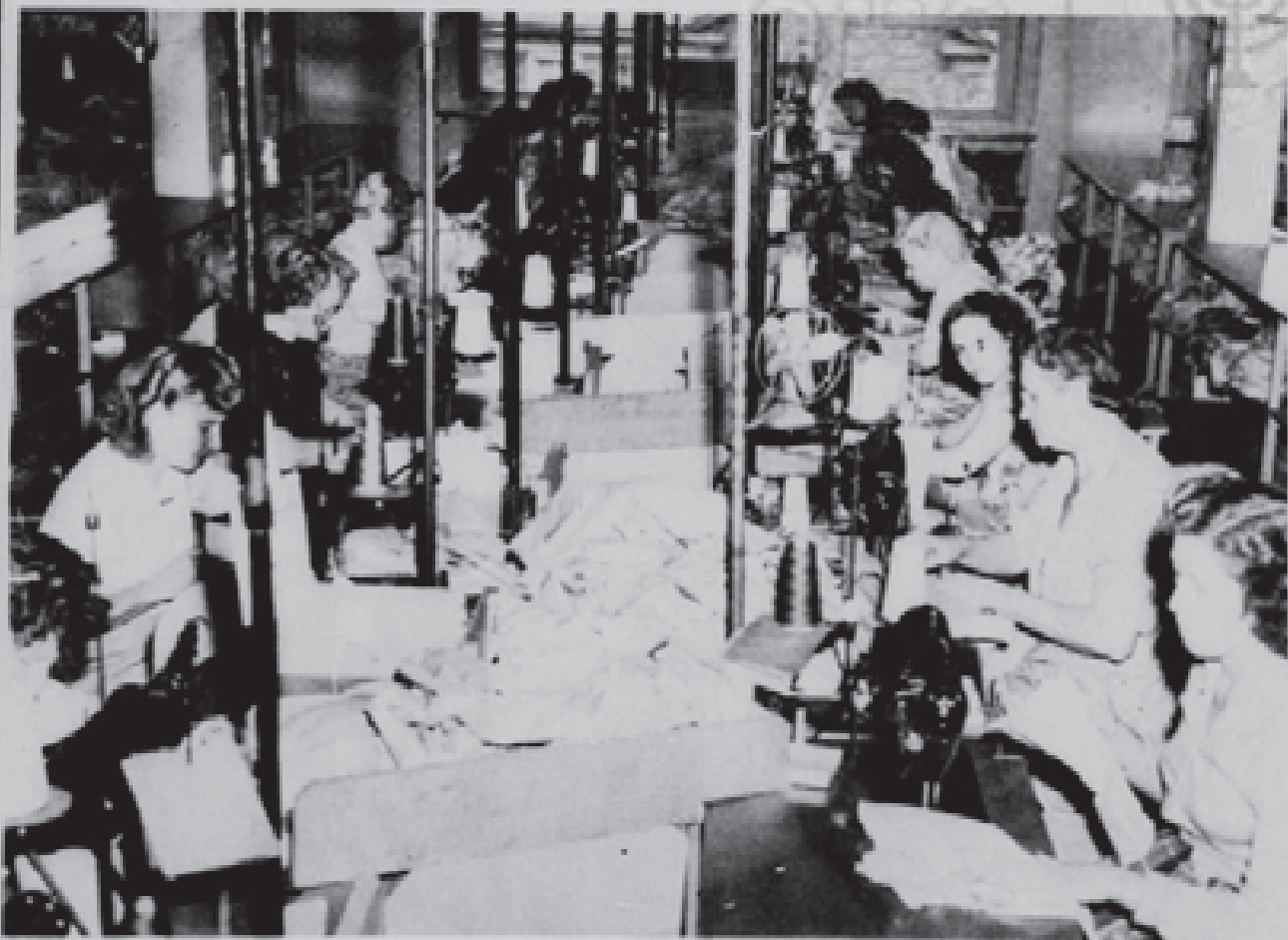
By setting the machines the width of the factory, we were able to increase our aisle space 12" and the storage bins between the machines from 16" in width to 18". (Pictures 1 and 2)
