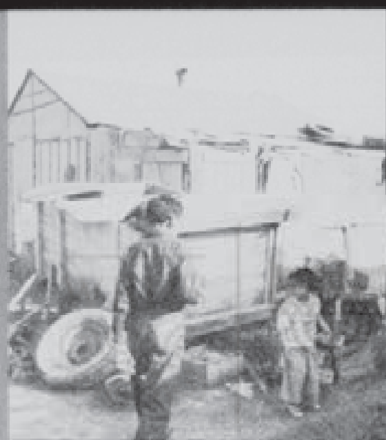
Migrant labor camp. Houses patched together from old scrap lumber and sheet iron, wet and cold in rainy weather.
