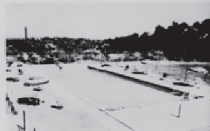
FILTERED OLYMPIC SWIMMING POOL
