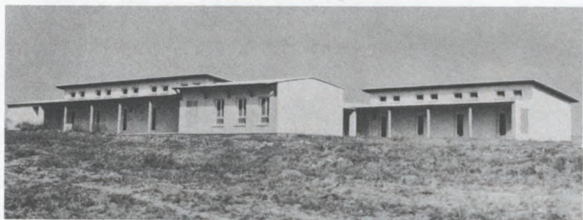
KFAR SILVER, Dormitory Buildings
