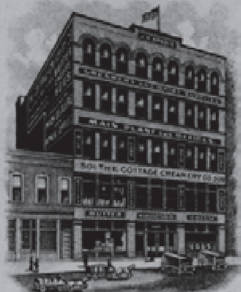
OUR OWN REFRIGERATING PLANT.
