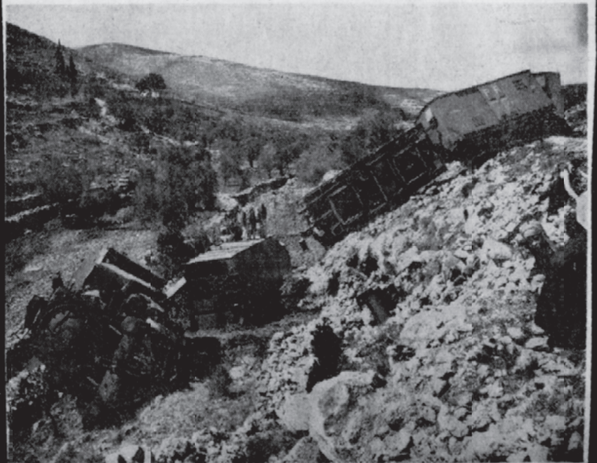
Wreckage of a freight train, derailed by explosives placed on the tracks, is strewn along the embankment near the Arab village of Beit Safafa, five miles south of Jerusalem
